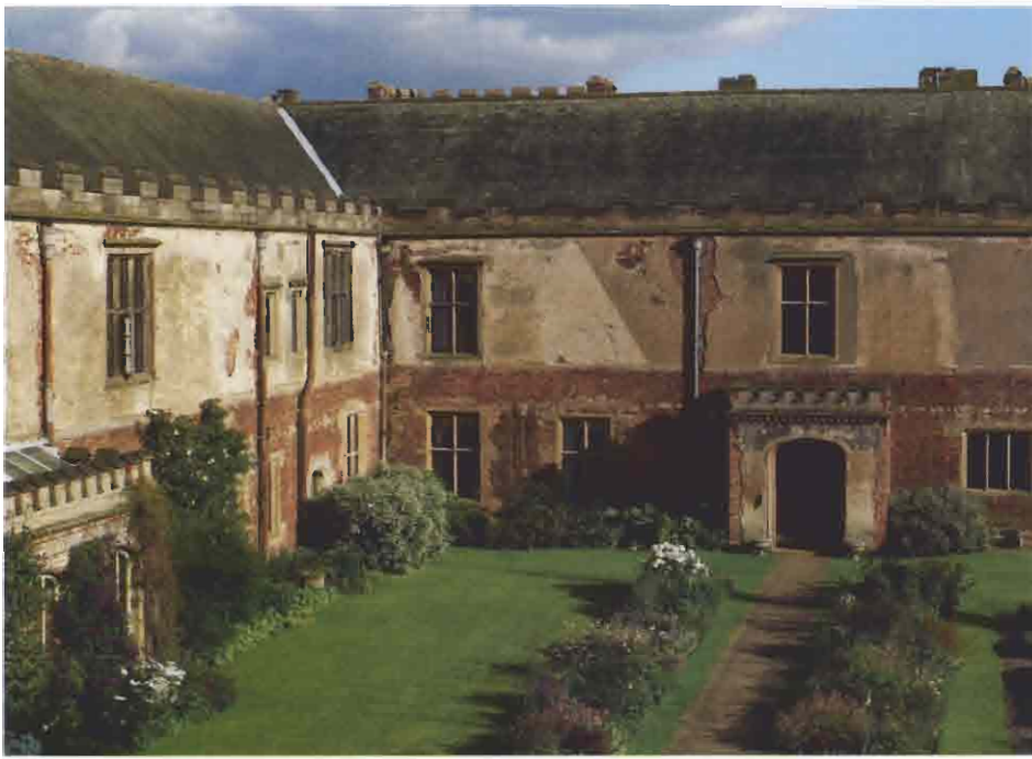
6—The courtyard, which originally featured a cloister, now contains a charming formal garden, the design of which is based on a late-19th-century layout. Surrounded on three sides by the house and on the west side by a fine battlemented wall, the garden feels both enclosed from, and connected to, the external Nottinghamshire landscape
