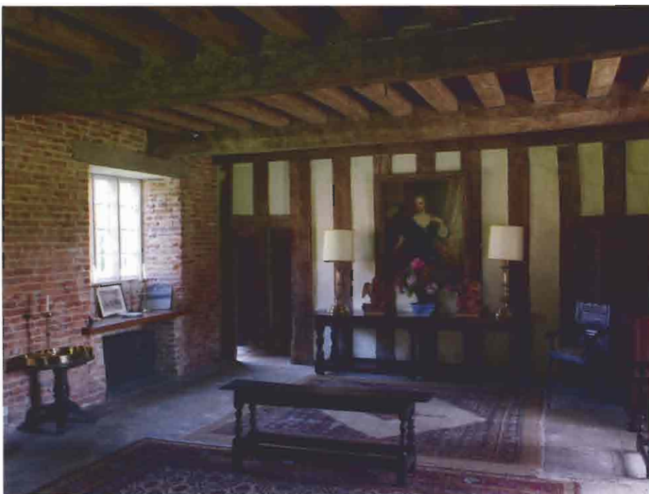
7—The spacious ‘lower lodging’, with its closely studded timber walls. Grandly proportioned, this interior is an appropriate and atmospheric space in which to perform official ceremonies such as marriages—all part of the new life of the house
