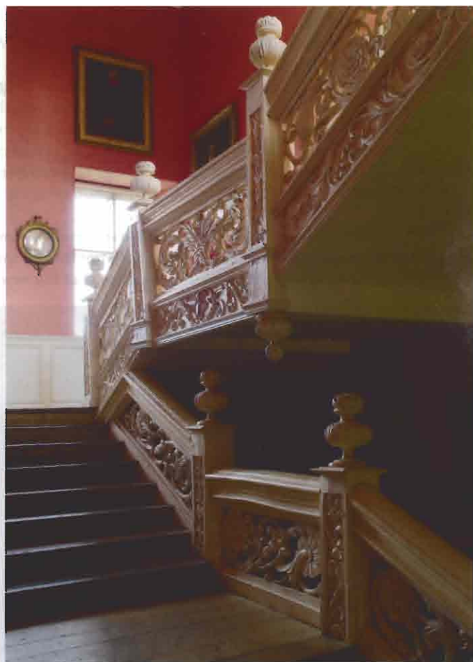
5—The 1660s oak staircase with its rich foliated balustrade and newel-post urns with carved fruit is similar to staircases at Sudbury Hall in Derbyshire, and nearby Thrumpton Hall. As at Sudbury, a John Fowler paint scheme has been adopted, with the joinery painted white. Here, the paint helps disguise the many repairs and reinstatements made during restoration in the 1970s
